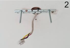
The big strip fastener is shown here being fixed to a standard flat ceiling. Using flat head screws, fix the big strip fastener using as many fixing screws as you can.
