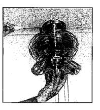
Take the weight of the fan and offer the canopy up to the mounting plate. Two keyed slots in the canopy will align with the two screws that have been left in the mounting plate.
