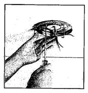
The mounting plate should be screwed on to a firm flat surface. The fixing location must be able to withstand ten times the static weight of the fan. If you have any doubts as to the ability of your intended fixing location to be able to withstand this loading please contact our service help-line or another competent authority to advise you. In most situation four wood screws screwed in to a wooden joist is more than adequate to support your ceiling fan
